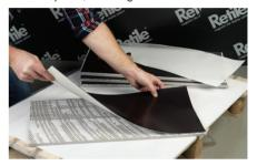
**6.** Position the Retile Magnetic Panel over the tile back and press down.
