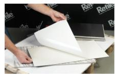
**5.** The Retile Magnetic Panels are supplied pre-cut to your specified size. Peel back the release liner to expose the special high bond adhesive.
