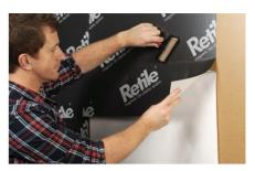
Peel back the release liner a little way and start to apply to the sealed substrate. Use the Retile Application Roll to apply pressure to the panel, ensuring no air bulbs.
