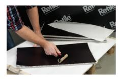
Start with a clean, flat substrate and seal it with a suitable primer and leave it to dry.
