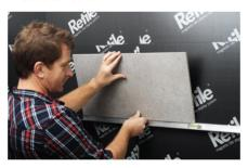
Using a spirit level to level up and place your tile with magnet on to the wall, and away you go.
