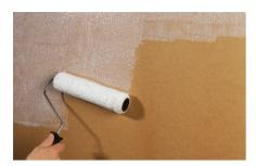
**1.** Start with a clean, flat substrate and seal it with a suitable primer and leave it to dry.
