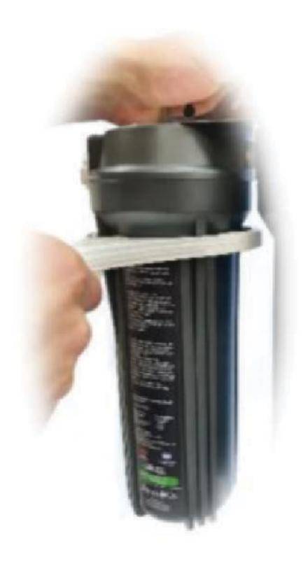
17. TIGHTEN HOUSINGS, FITTINGS OR CONNECTIONS - If tightening doesn't stop the leak, you may need to replace the faulty component or fitting, or consider using plumber's tape for threaded connections.
