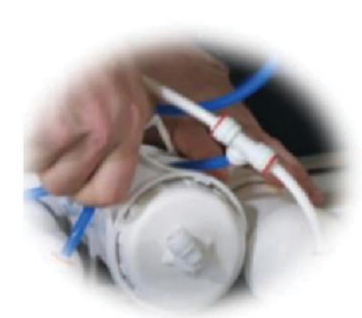
11. CLOSE HOUSING CAP - Screw in the membrane housing cap by hand and locate your membrane spanner to tighten it.
